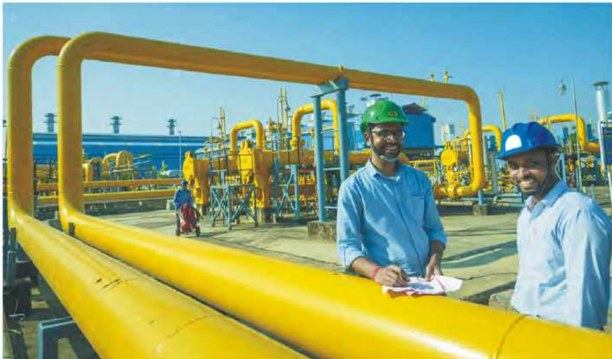
GAIL Engineers at work at Plant
